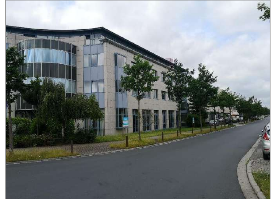
R&D Office, Germany
